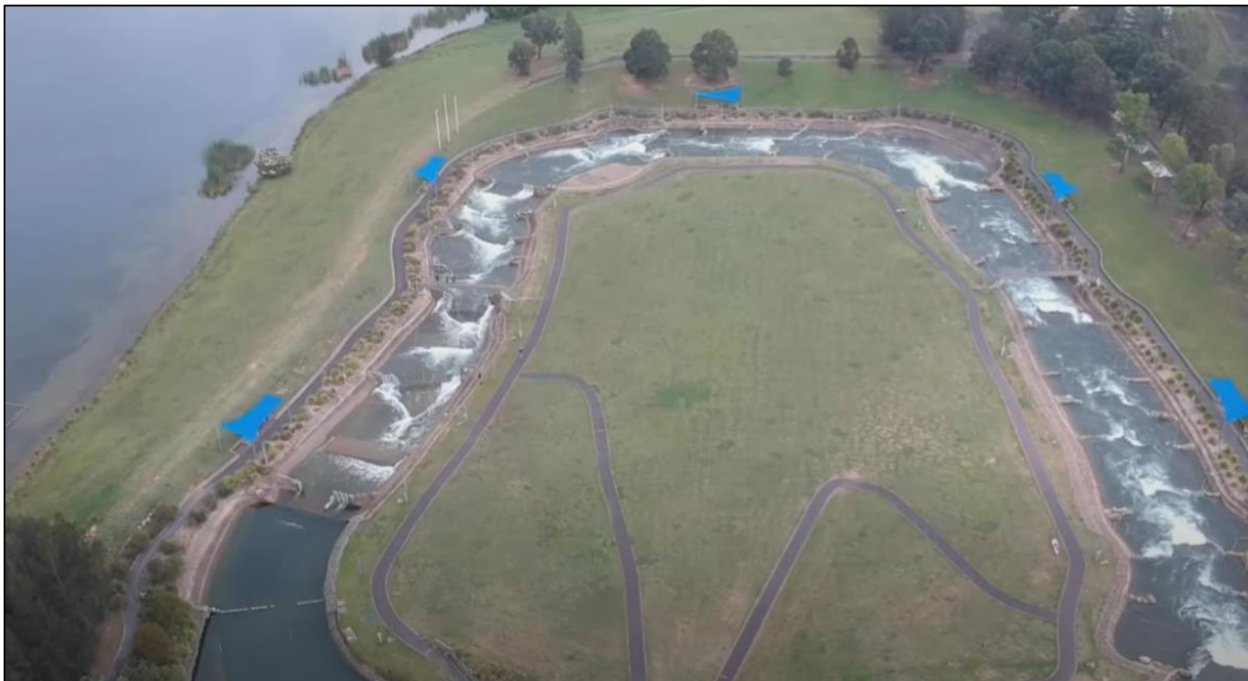
Figure 14 Aerial view of Penrith Whitewater Stadium
