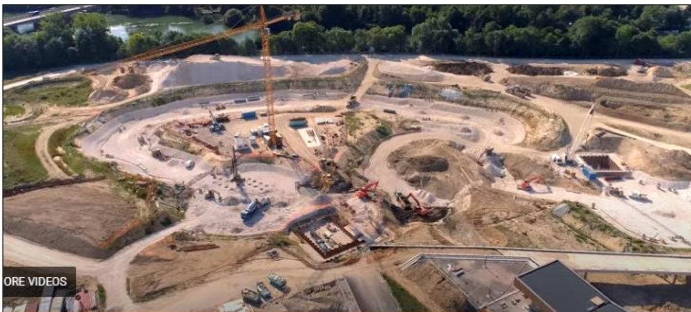
Figure 5 Paris 2024 Whitewater venue under construction
